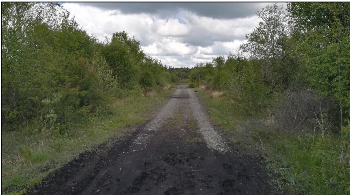
Plate 12-16 Established vegetation along an access track.
